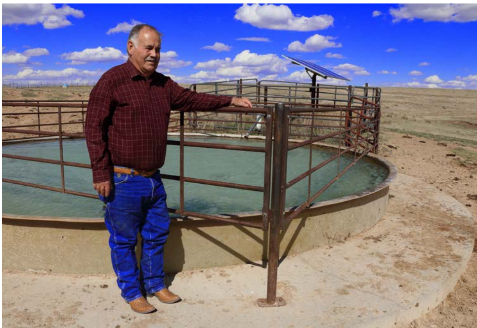
The Panhandle rancher has installed solar-powered wells to water livestock. He uses two panels to power a 1 horsepower pump, drawing water from about 120-feet below ground.
